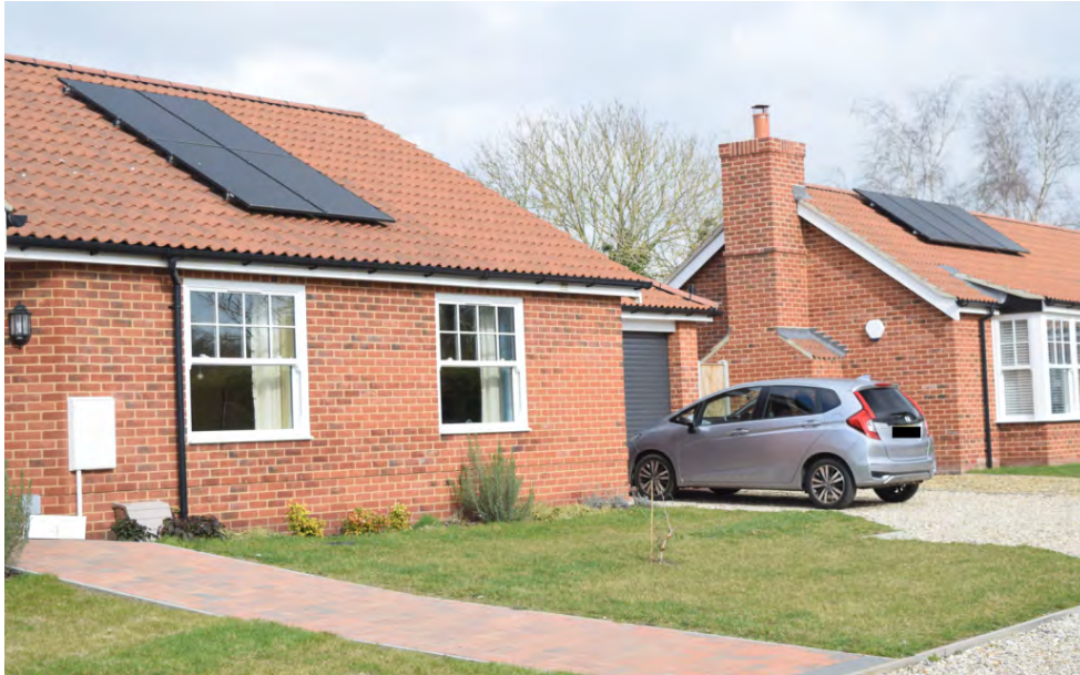
Figure 4: Examples of Energy Efficient Technologies (Source: AECOM Design Codes and Guide Document, 2022)
