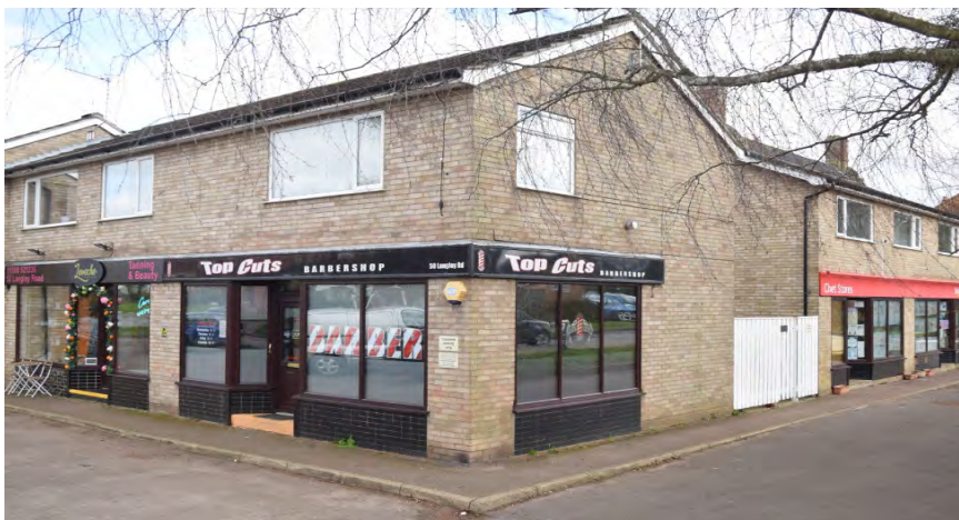
Photos of part of Chedgrave’s Shopping Strip
