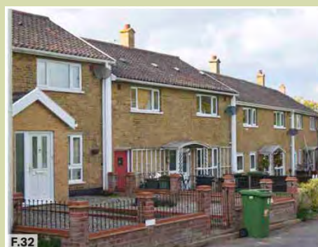
Figure 32: 2 storey terraced housing designed by Tayler and Green.
